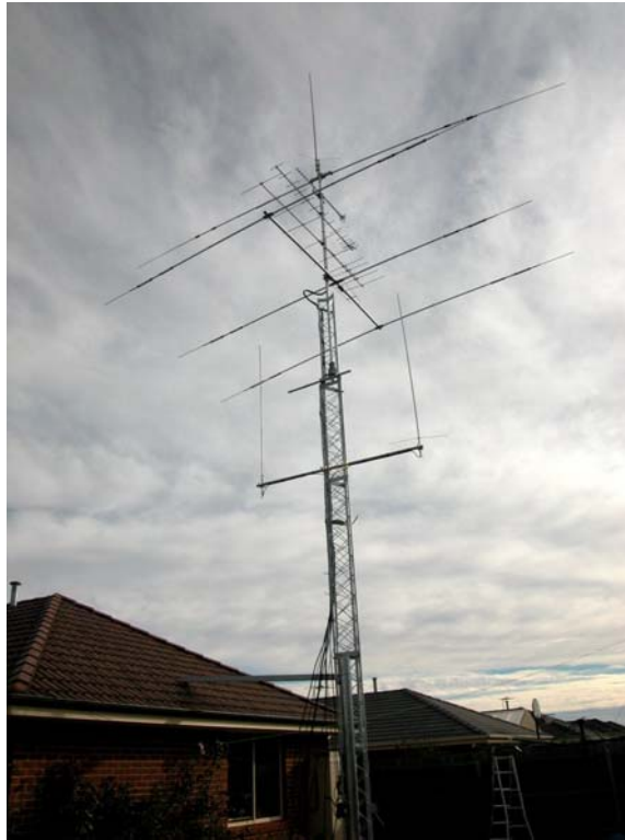
Photo of the new VK3UR antenna farm, prior to installation of the cables (and speaker wires) in the roof and slight straightening of a few elements.
